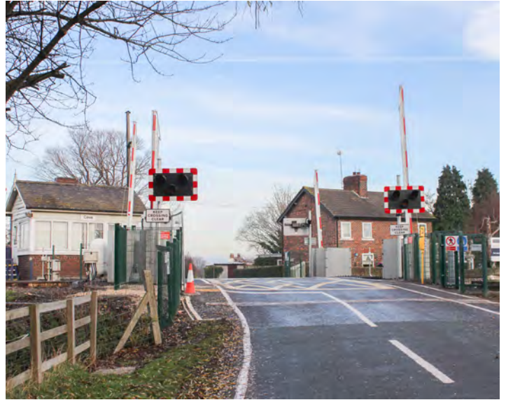
Cave Crossing gate box has been replaced with Cave obstacle detection crossing. Photo Network Rail.
