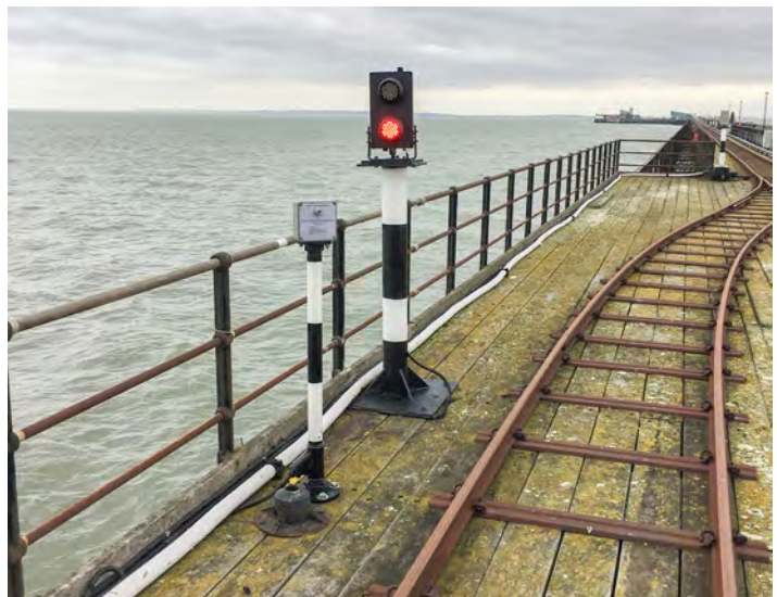
South end exit of the loop showing refurbished treadle D2, new key-switch post T2 and new Dorman LED signal head (L2) on the refurbished post.
