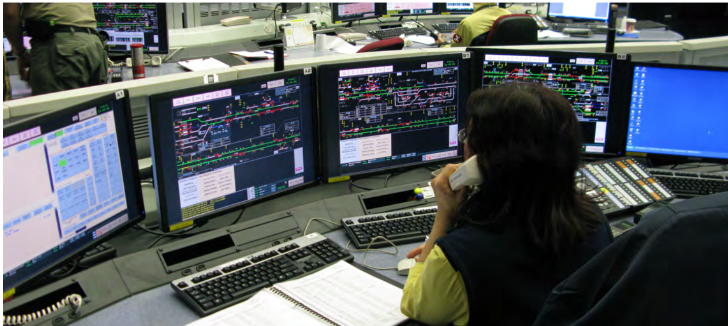
Figure 9 – The use of computer-based interlocking, and increasingly the use of network communications, allows modern control systems to be implemented, as in this example from Hong Kong MTR. The interlocking continues to ensure that the signalling rules are enforced to assure safety, but the non-vital control system above allows the railway to be operated optimally. Photo Francis How.
