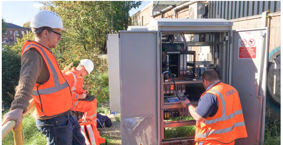
All trackside equipment is contained in a smaller number of location cubicles with no equipment buildings required, thus saving both cost and space.
