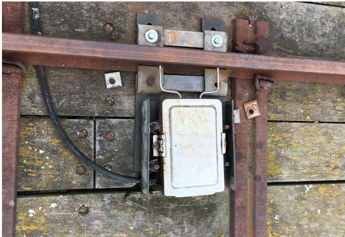
Installing the refurbished treadle (D2).
