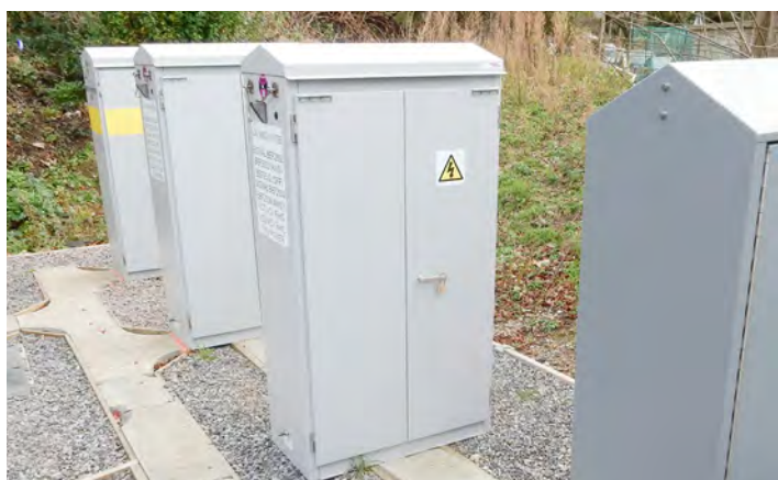
Top left: Far left are two control centre cubicles, coloured red and yellow, and to the right Multi Service Network (MSN) interlocking and MCB-CCTV cubicles.
