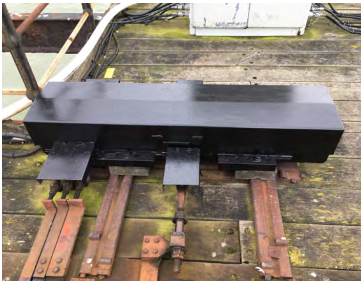
Refurbished point machine cover for points P1 at the north end of the loop.
