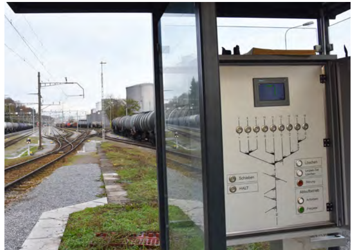
The re-signalled, nine-track Auhausen hump in 2019 and its new local control panel, which an operator can use wearing gloves. Photo George Raymond.
