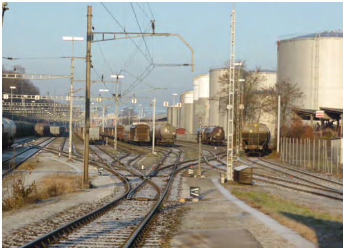
The nine-track Auhausen hump yard in 2013, before re-signalling. The project removed the connection between tracks 4 and 5 and renumbered all tracks. Photo Bruno Huber.
