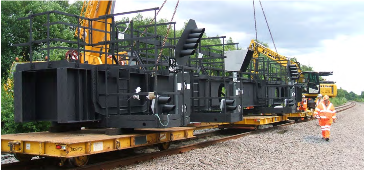
Gantry P2 at Tapton, near Chesterfield, being moved to site. A case of true 'road and rail' movement.
