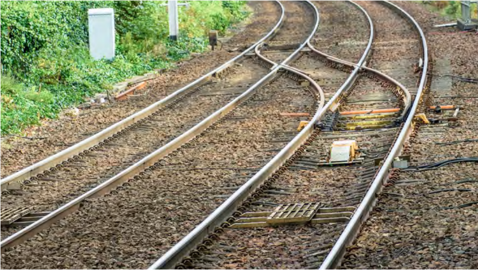
AWS (the yellow magnet middle right of the photograph) and TPWS (right foreground) still work together across the UK rail network. Photo Shutterstock/TreasureGalore.
