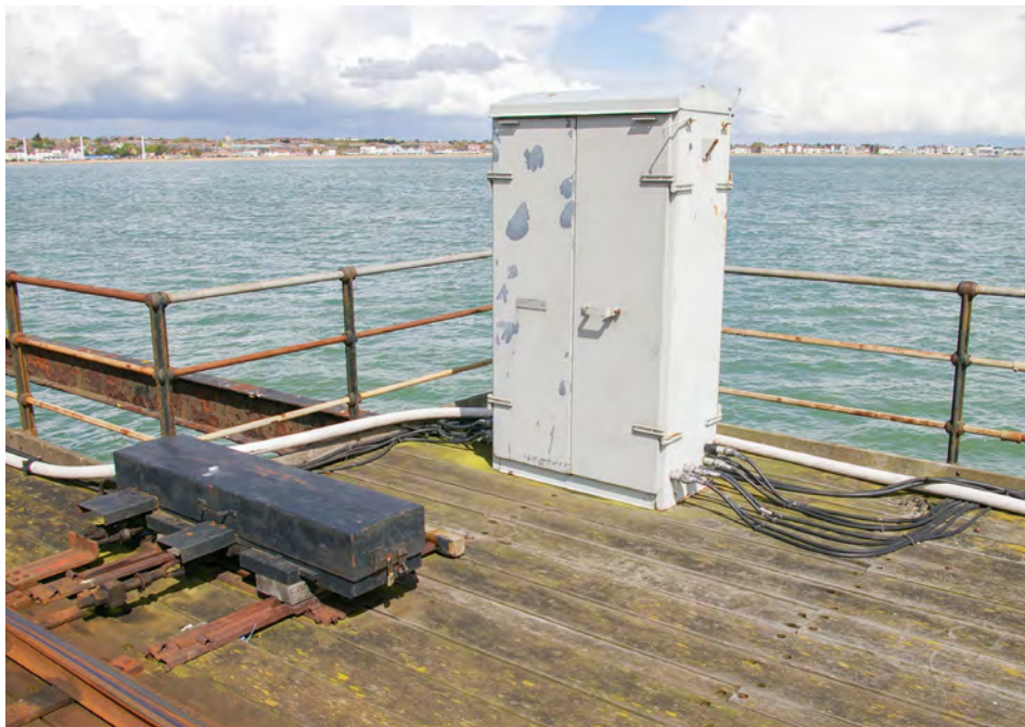
Location case and HW1121 point machine before refurbishment. The high tide on the day when this photograph was taken gives an impression of how exposed to the elements the equipment is.
